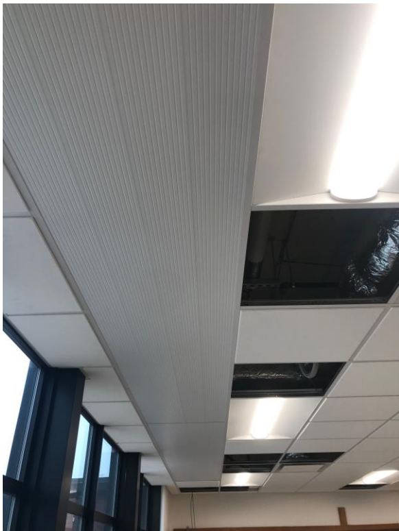
Ceiling Radiant Panel
